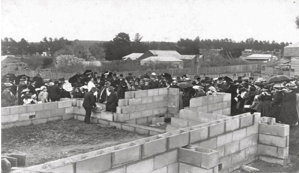
The ceremony of the laying of the foundation stone at the Parish Hall in 1909. The innovative construction method, using concrete blocks and no frame, can be clearly seen in this photograph. Photo: LDHS archives
