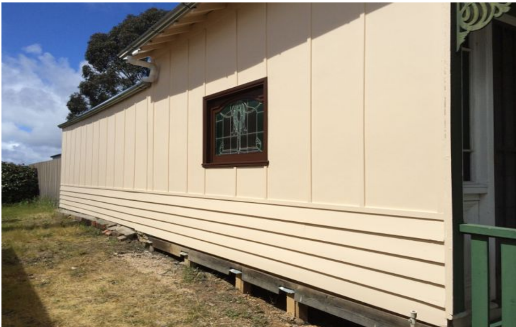
Since Jill's report to the AGM, the proposed works she mentioned have been completed. Here is the new wall at the Nelsons' Undertakers' building painted in heritage colours. The work was carried out by James Overton of Linton.
